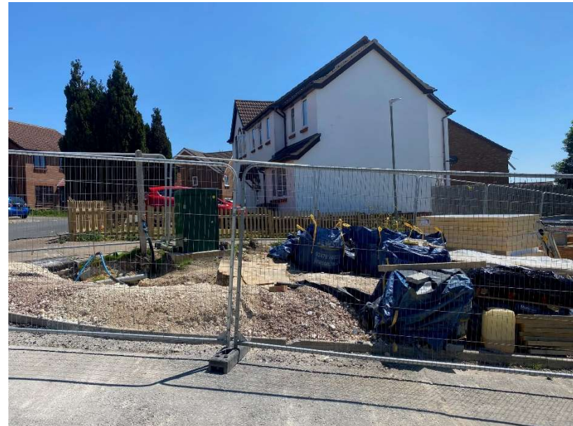
After commencement of construction (10/6/21)
